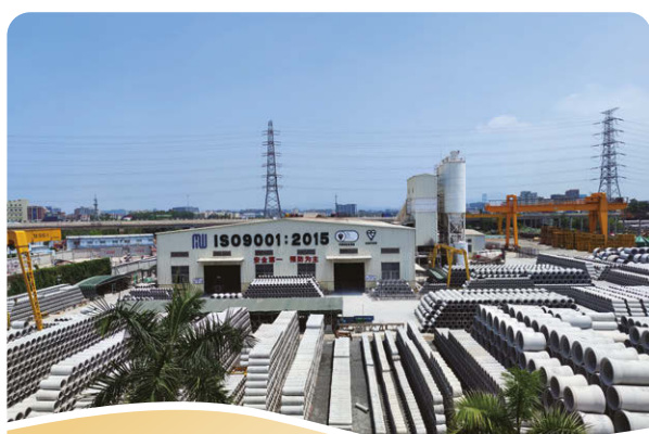
Concrete precast factory located at Shajing, Shenzhen
