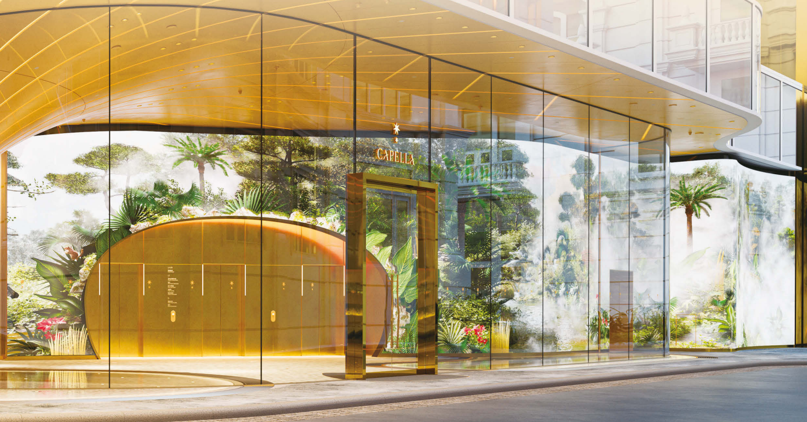
Capella at Galaxy Macau Entrance Driveway
