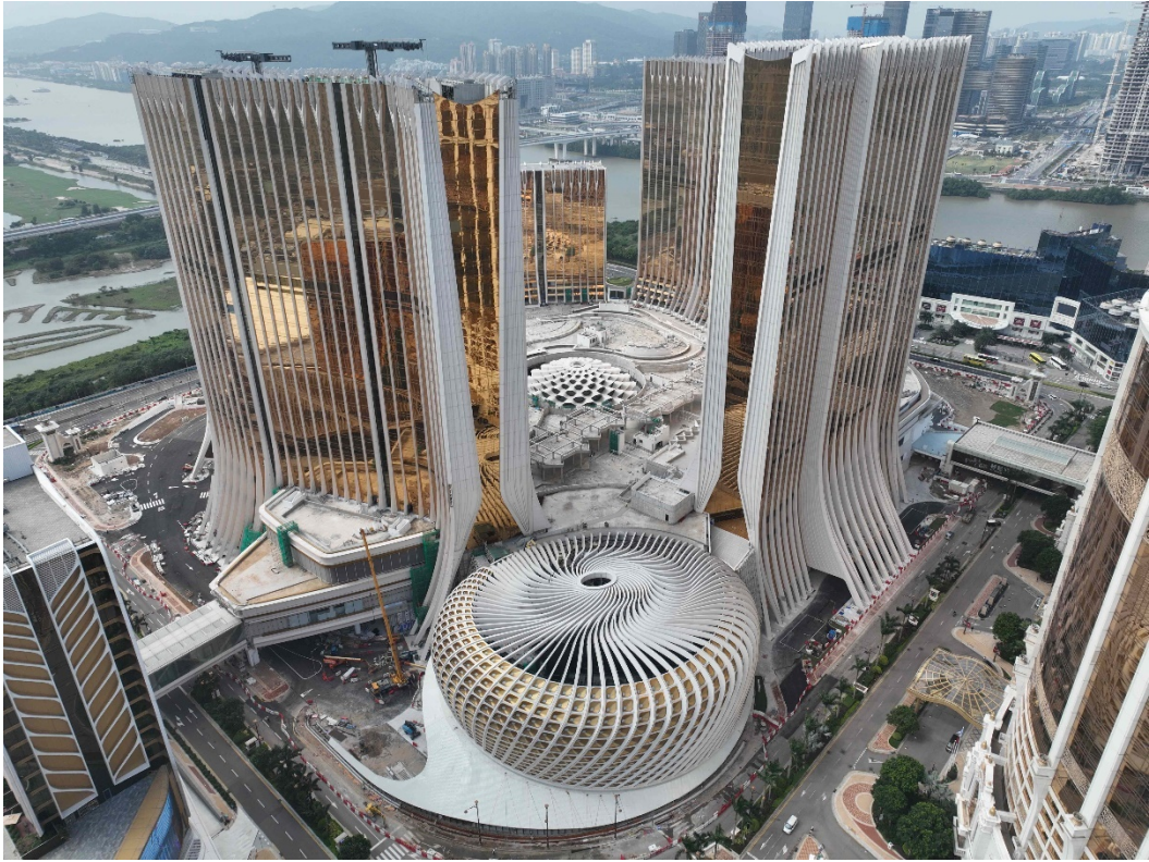
Latest photo of Cotai Phase 4 (November 2024)
